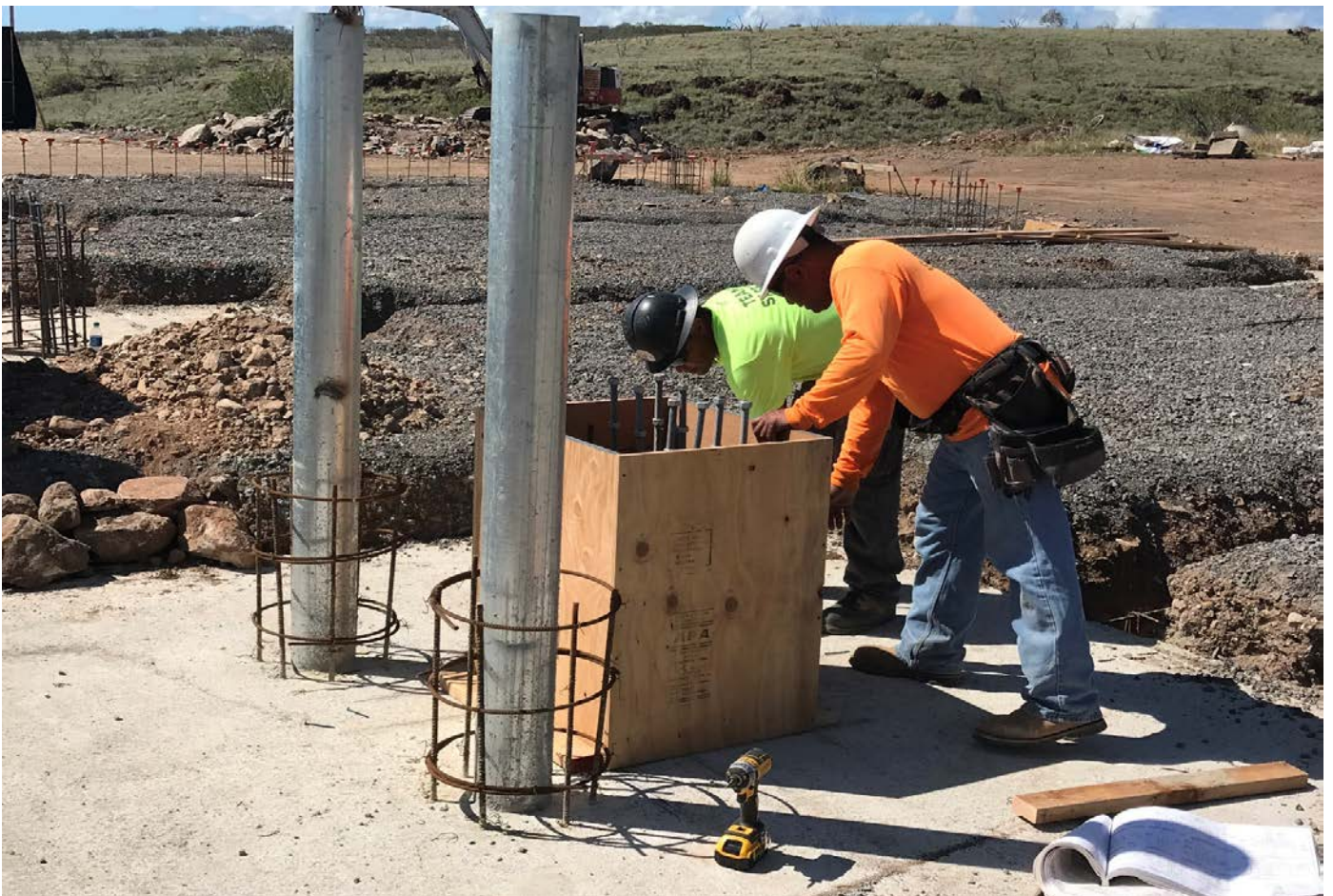
Molokai Baseyard Facility
