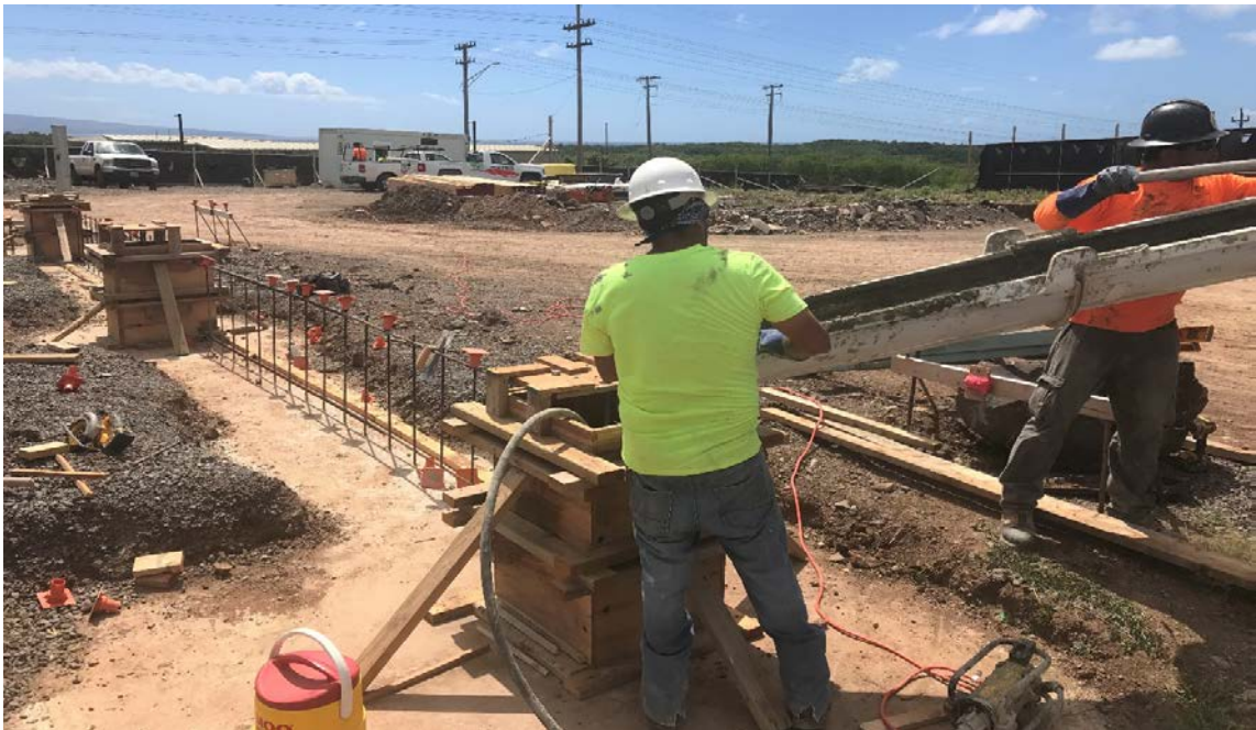
Molokai Baseyard Facility
