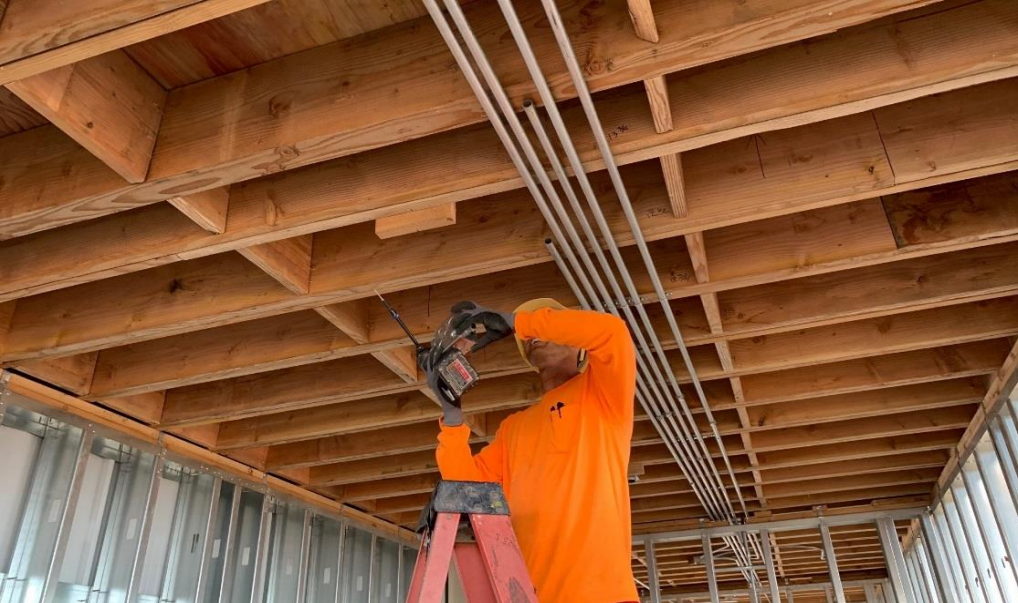
Molokai Baseyard Facility
