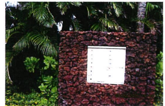
Custom Box installed by Developer
