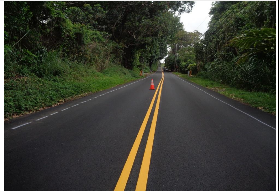
DSC00102 – Centerline pavement striping.
