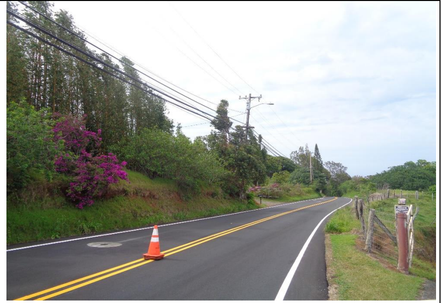
DSC00043 – Edge and Centerline striping
