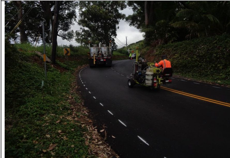
DSC00101 – Double centerline striping with buggy.
