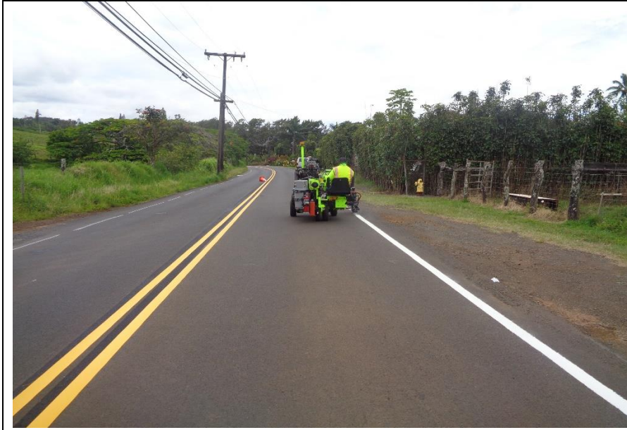
DSC00037 – Edge striping with buggy
