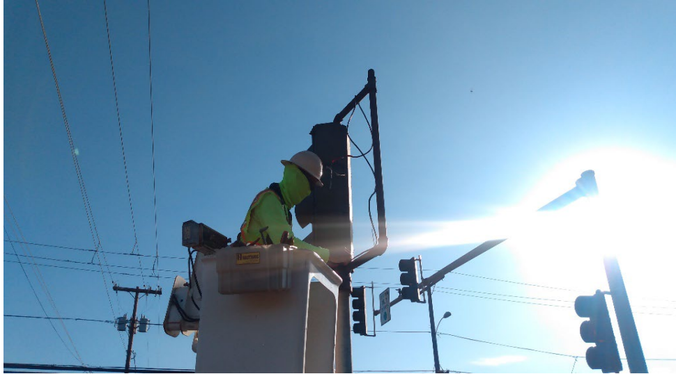
Installing Microwave Camera
