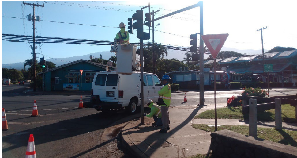
Installing Microwave Camera
