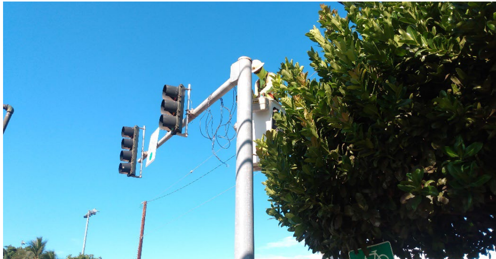
Installing Camera on Traffic Arm S. Kihei Rd.
