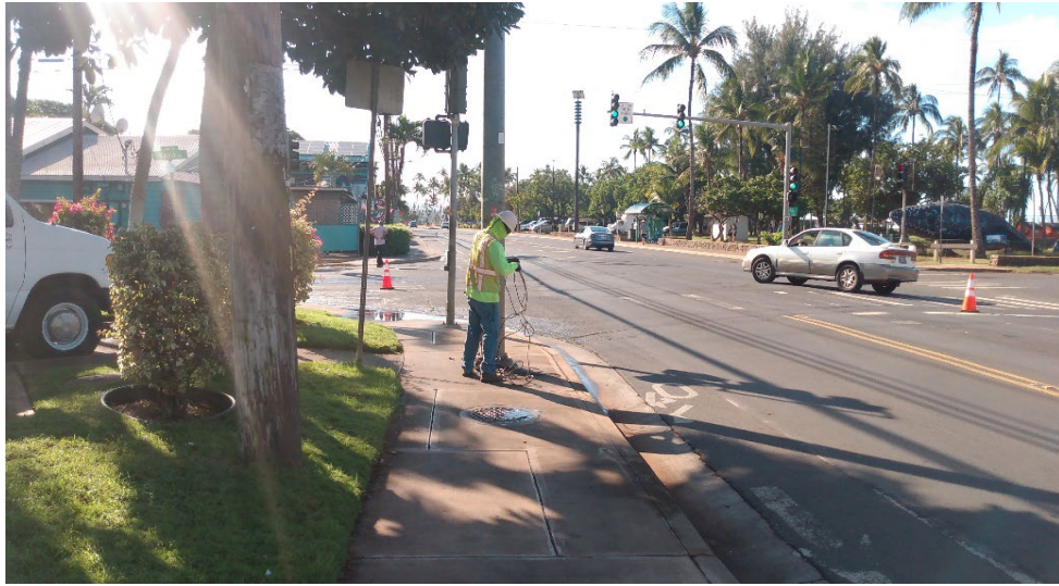
Installing Traffic Camera
