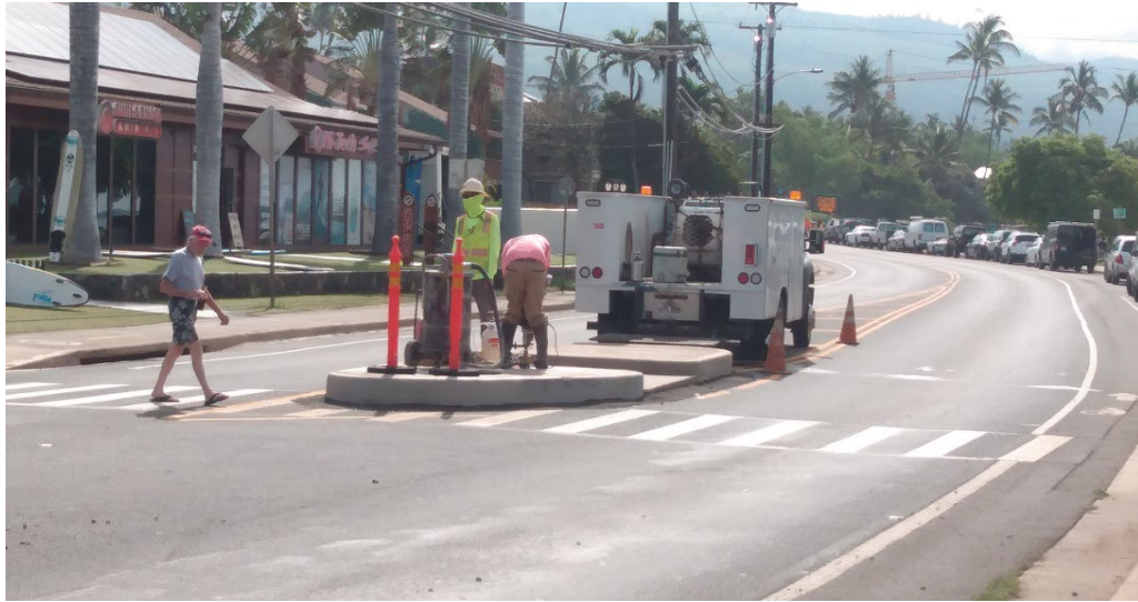
Coring for RRFB at Crosswalk at Auhana Rd.
