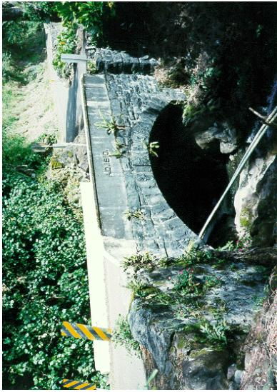
Preliminary Recommendation: **Preserve makai facing of arch and rail. Construct new slab over existing bridge.**
